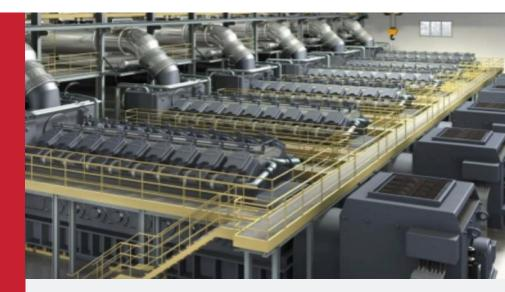
The facility will generate electricity at the 13.8kV level before increasing to 138kV, where it will be connected in parallel to the provincial grid and subsequently fed to the mine site.
